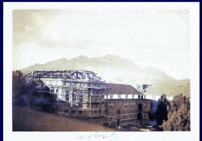
The construction of the dining hall in August 1927
